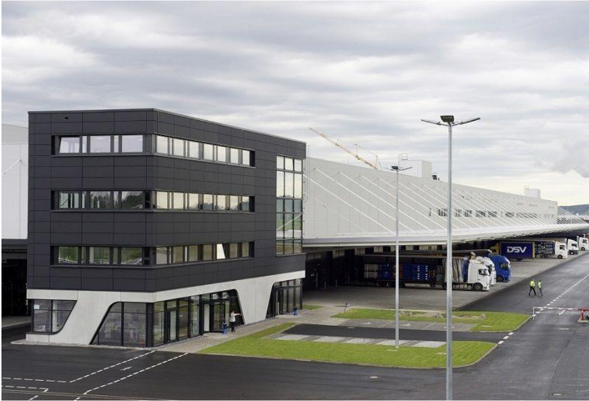
The Böllinger Höfe site is equipped with particularly energy-saving LED technology.
