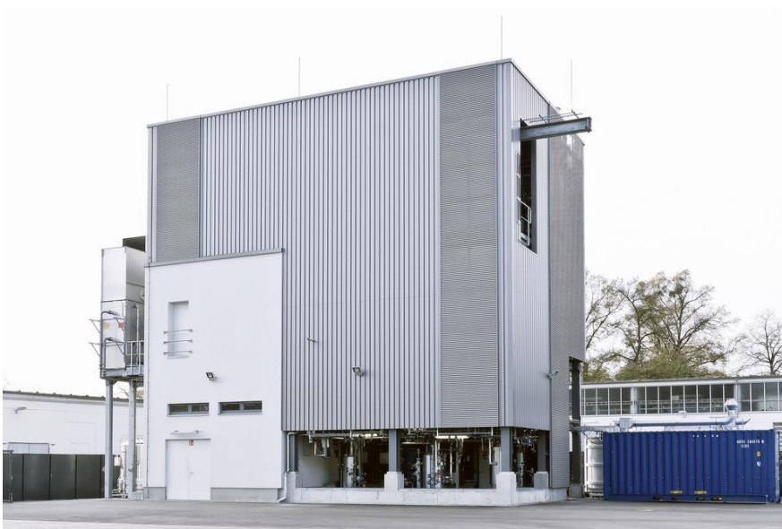
The sunfire plant in Dresden produces Audi e-diesel from carbon dioxide, water and green electricity.
