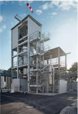
In the methanation unit (centre picture), the hydrogen is converted into synthetic methane by adding CO<sub>2</sub>.
